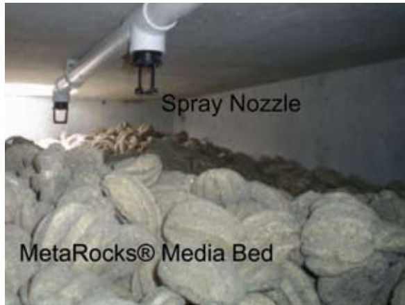
View Inside Eliminite showing MetaRocks and spray nozzle
